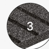
GROOVE WITH EPOXY FILLING
